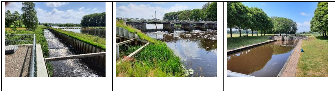
Figure 16: Fish ladder (left), weir (centre) and navigation sluice (right) on the Vechte River (pictures Marnix van der Vat)
